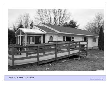
Leger House - USA – 1977 Double wall – R 40 walls R 60 ceiling Airtight construction Air to air heat exchanger
