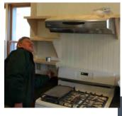
Sealed combustion, mechanical ventilation w/ HR, spot ventilation, reduced mold - no cold condensing surfaces
