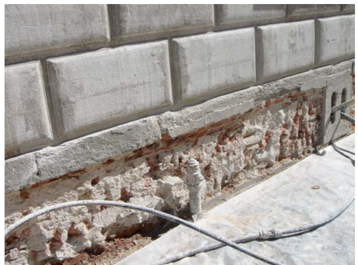
Photograph 3: Sacrificial layer being applied in Prague, Czech Republic
