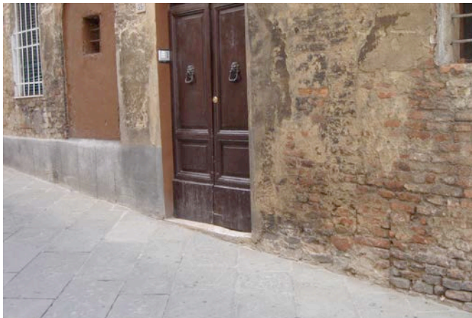
Photograph 4: New sacrificial layer in Firenze, Italy
