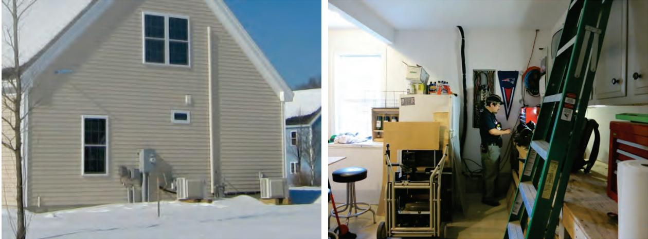
**Figure 79. Retrofitted unit and line set for second-floor MSHP on exterior (L), and in garage (R)**
