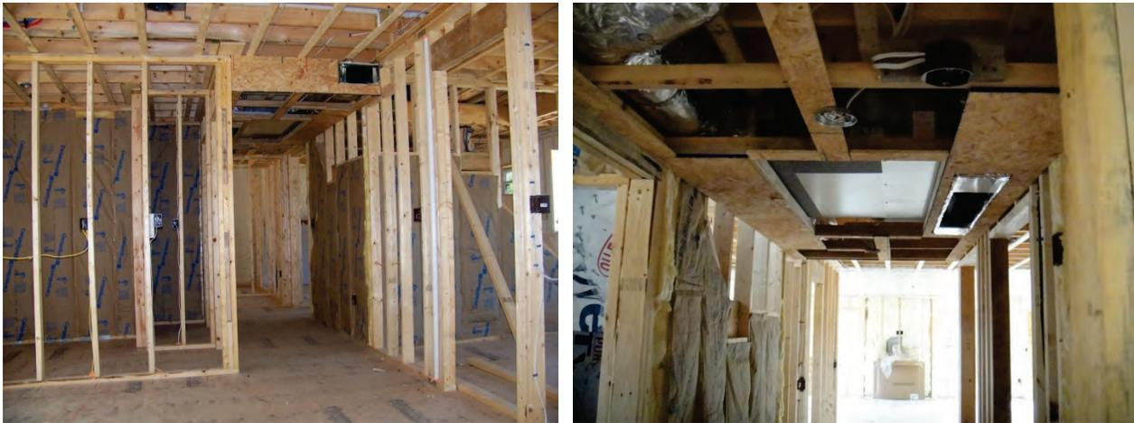
**Figure 10. Ducted air handler MSHP indoor unit, at Transformations’ Townsend development**
