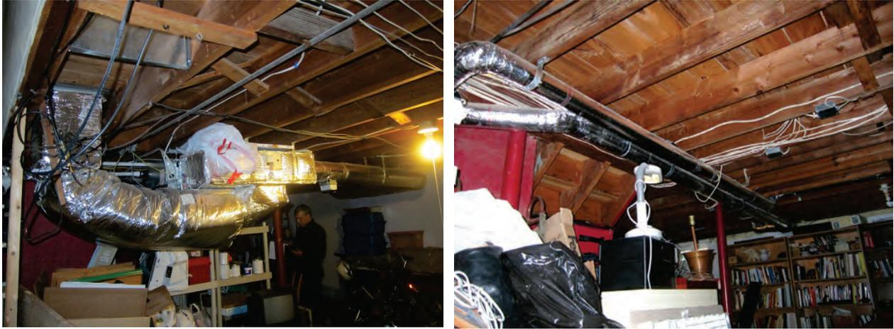
**Figure 11. Ducted air handler MSHP indoor unit, with excessively long/restrictive ductwork**
