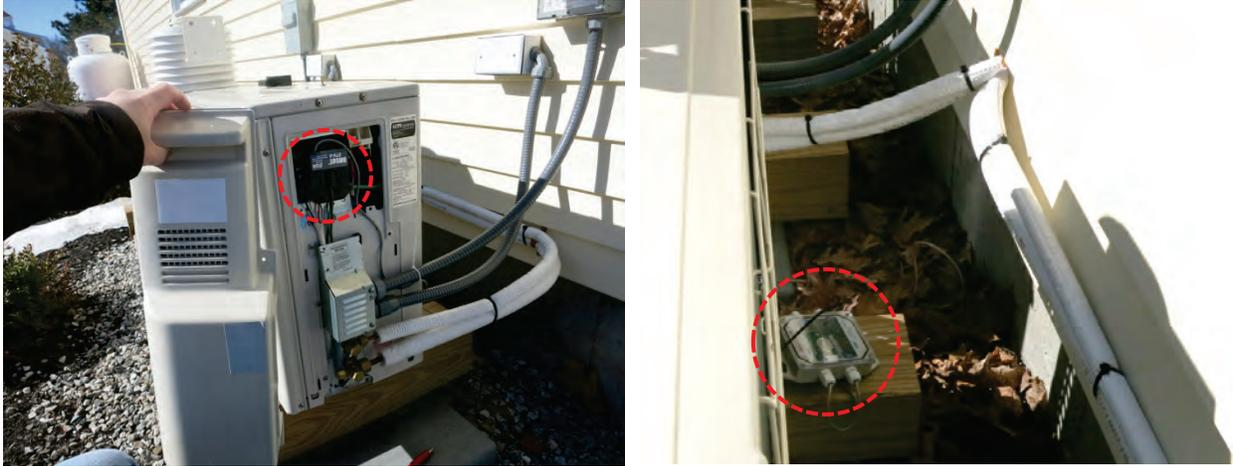
**Figure 18. MSHP electrical power monitoring at outdoor unit**
