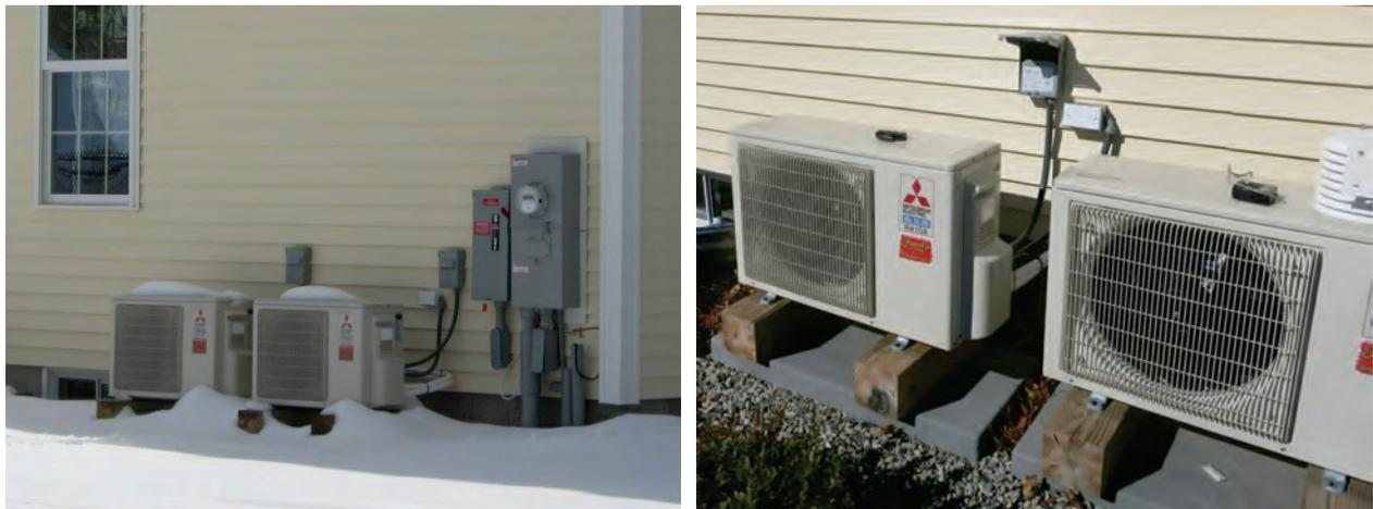
Figure 34. Outdoor units raised on wood block risers
