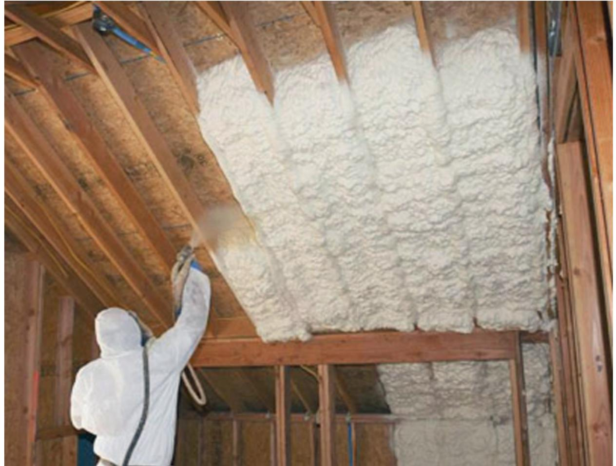
Except that open-cell spray foam is associated with damp roof sheathing...
