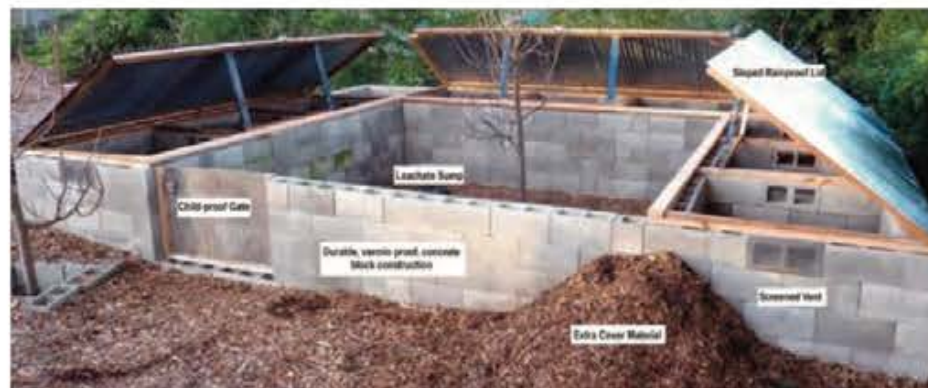
Compost bin system at Kailash Ecovillage in Portland, Oregon with child-proof gate, screened vents, and durable concrete blocks to prevent animals from getting in. Credit: Ole Ersson in The Compost Toilet Handbook
