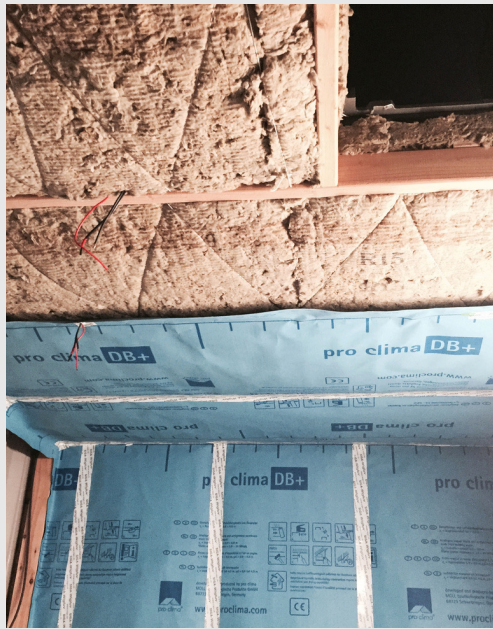
CONTINUOUS, TBF INSULATION
