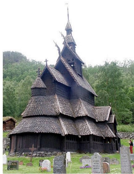
Photograph 1: Stave Church— Borgund, Laerdal, Norway, 12 th Century. Image taken by Frode Inge Helland.
