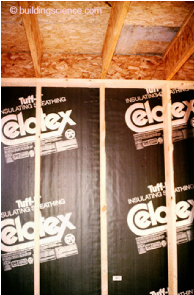
Photograph 5: Building America —Advanced frame 2x6 structure, studs on 24 inch centers, single top and bottom plates, 1.5 inches foil-faced polyisocyanurate insulating sheathing. Cavity insulation not yet installed. This is likely to be the industry standard in the next decade. R&D courtesy of the US DOE Building America Program.
