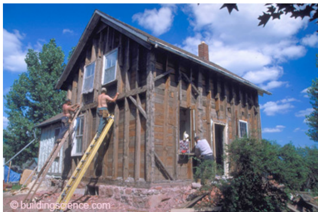
Photograph 2: Exposed Timber Frame —One hundred and fifty year timber frame house being renovated. Exterior horizontal sheathing boards and weatherboards removed. Note the close spacing of the vertical intermediate posts.
