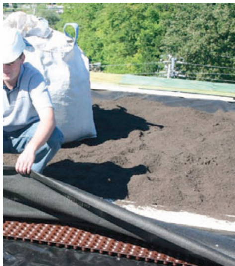
Photograph 4 (above left): Root Barrier and Drainage Layer —Both are a big deal. Notice the filter fabric above the drainage mat and the root barrier under it. Figure 4 (above right): Green Roof —To turn a PMR or IRMA into a green roof, add a root barrier, a soil-based growth medium (a.k.a. “dirt”) and plantings (a.k.a. “grass”). Make sure that drainage occurs above and below the insulation layer.
