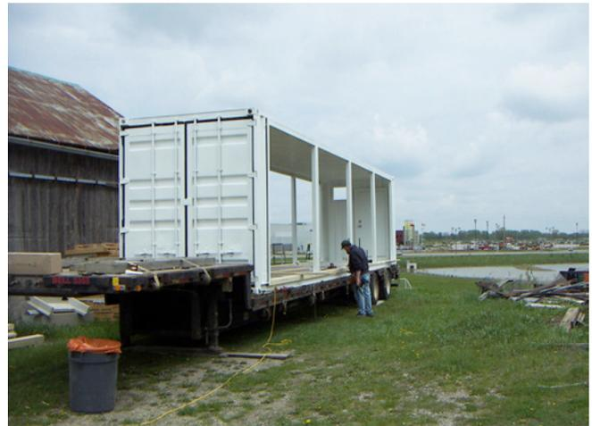
**Photograph 5: Adaptive Reuse** – The “building science research” version. This “test hut” was “anally” water and air sealed on the exterior and insulated on the interior with non water sensitive high-density (2 lb/ft<sup>3</sup>) spray polyurethane foam (SPF). Minimum of 2 inches of SPF yields a vapor transmission of less than 1 perm. You get a Class II vapor retarder, which means you can use this approach everywhere – even in Tuktoyaktuk.
