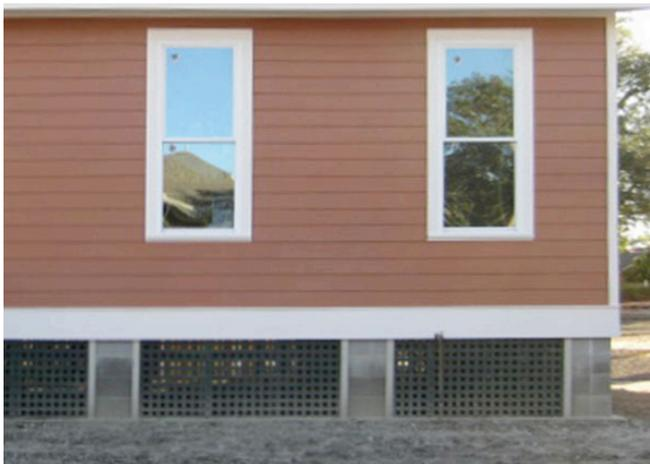
**Photograph 4: Elevate the Structure** – This works for mobile homes and for shipping containers. Lift them off the ground, insulate underneath them and screen the perimeter.
