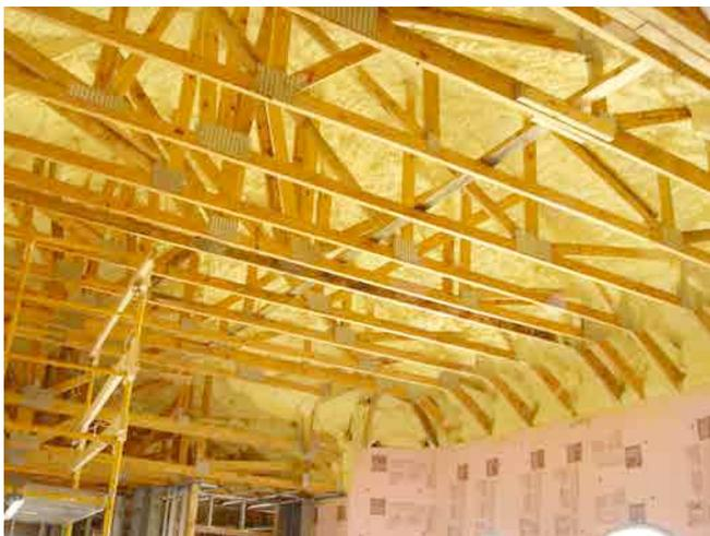
**Photograph 2: Open-cell Spray Polyurethane Foam (SPF)**—You cannot use open-cell in IECC climate zones 5 or higher unless the foam is used with a Class II (or Class I) vapor retarder. With open-cell foam a significant amount of moisture via vapor diffusion will pass upwards through it during cool periods and during the winter in cold climates—too much to be driven back down during sunny weather and
