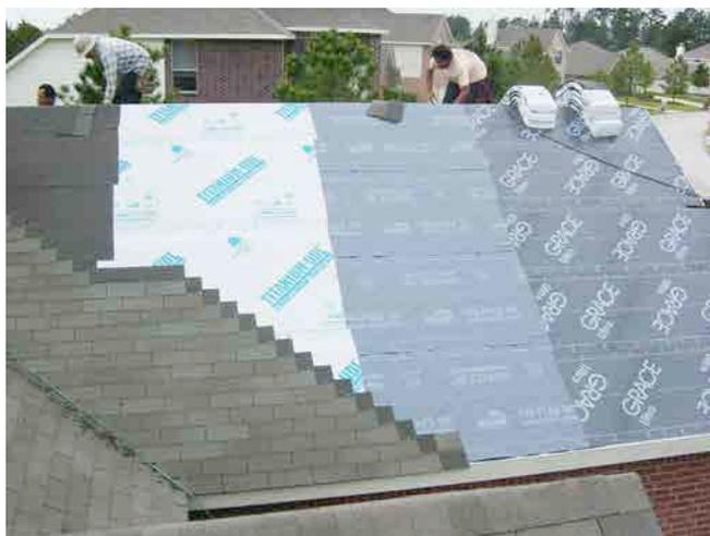
**Photograph 3: Test House in Houston, TX**—Back in the day some of us were worried about inward vapor drive through shingles into the roof deck in hot-humid climates. With an unvented assembly underneath there was some concern about the durability of the roof deck. At the time we had no idea how big the inward drive could be. We looked at it over a couple of years in test structures in hot-humid climates. It turned out not to be large enough to worry about.
