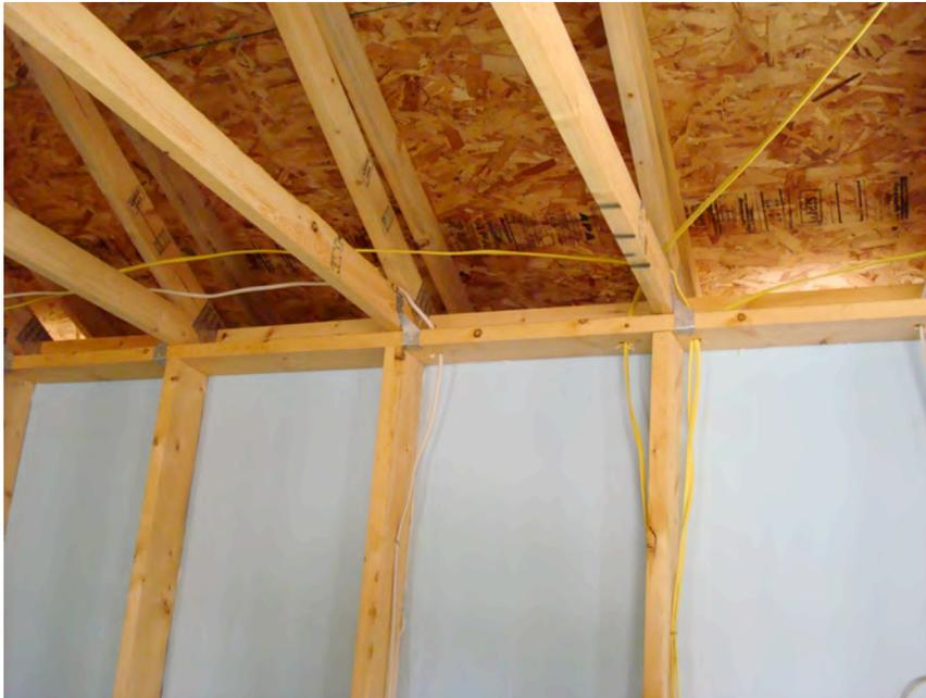
**Figure 3.3: Photograph of advanced framing showing single top plate and insulating sheathing**
