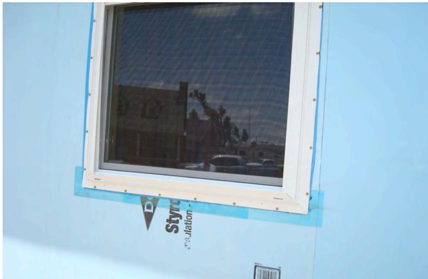
**Figure 3.4: Photograph of partially complete window flashing**
