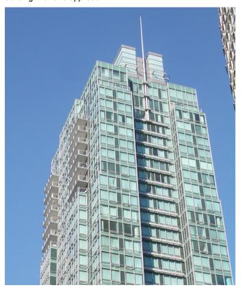
How should one choose glazing for green, low energy commercial buildings? At the most basic level, there are three critical measures of performance that must be chosen in design, and specified in contract documents: The U-value (1/R-value), the Solar Heat Gain Coefficient (SHGC) and the Visible Transmittance (VT).
