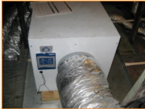
dehumidification through standard cooling during periods of high cooling. Initially, the 90 pint Aprilaire® Model 1750 dehumidifier's operation dial was set in the 3-5 range, per the manufacturer's installation manual. This was too high of a setting and it resulted in the dehumidifier running too much. The 90 pint unit outputs around ~10 kBtu while operating. This was
