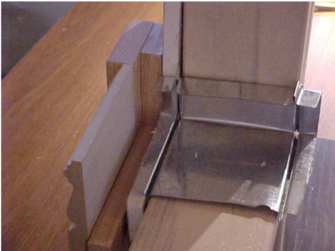
This picture clearly shows the air path behind the trim and the drywall detail.
