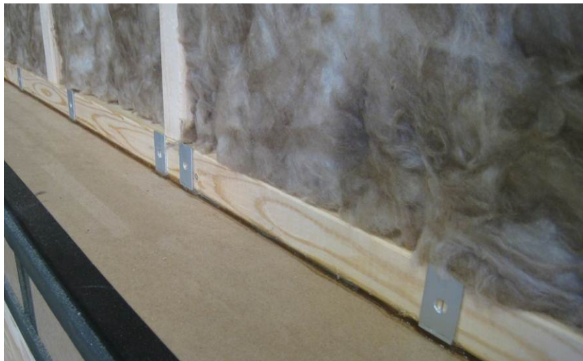
Figure 16 – Drywall Spacers and Fiber Glass Batt Installed
