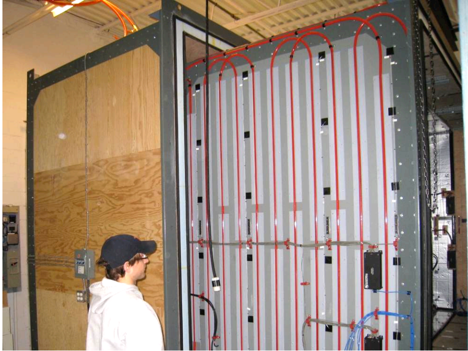
Figure 5 – Double Guard: Guard Box (Left) and Liquid Guard Loop on Meter Box (Right)
