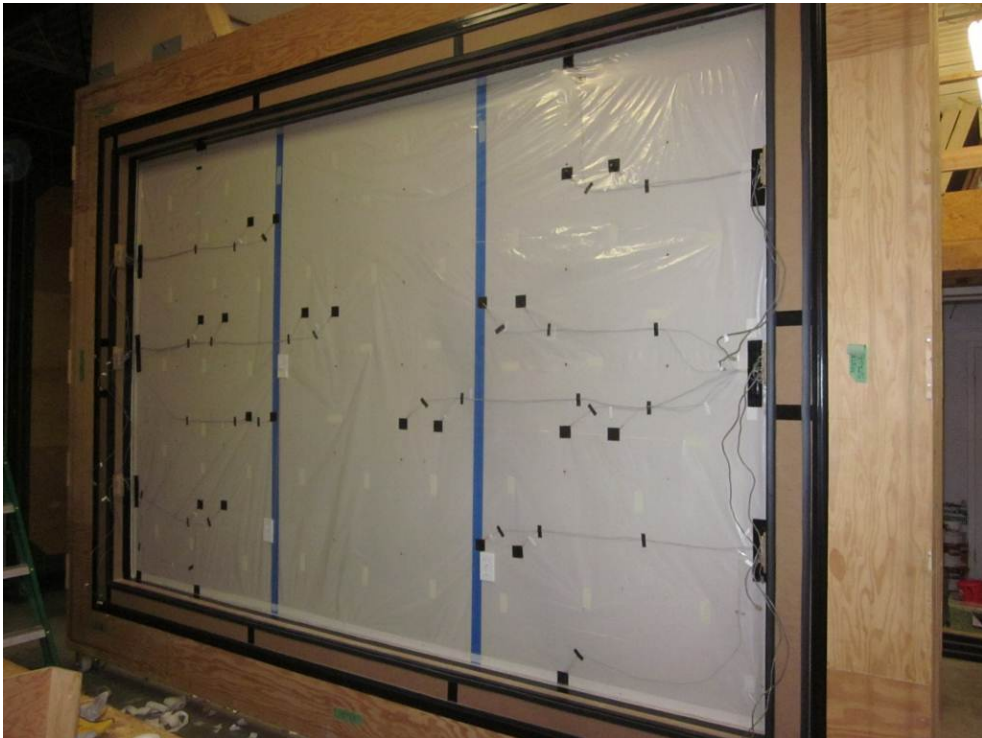
Figure 25 – Meter Box Side, Polyethylene Installed
