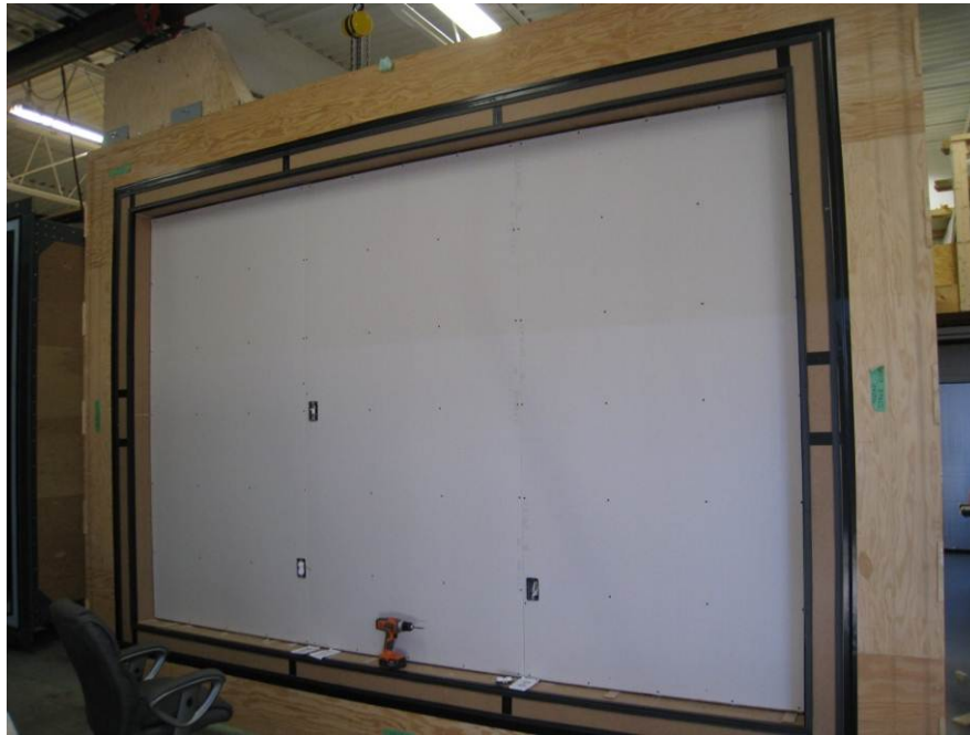
Figure 18 – Drywall Installed
