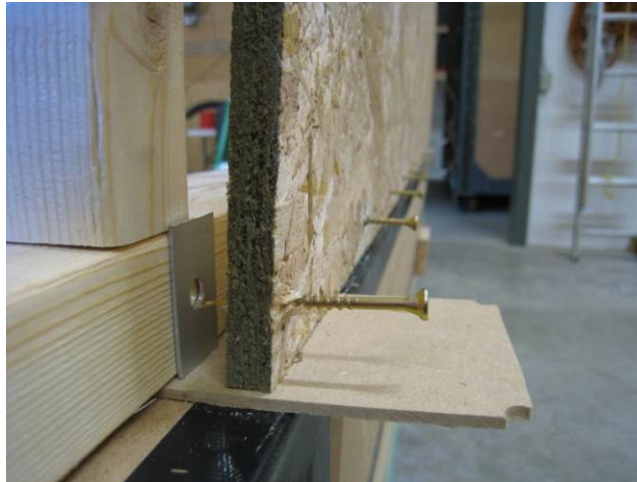
Figure 13 – Spacer Installation
