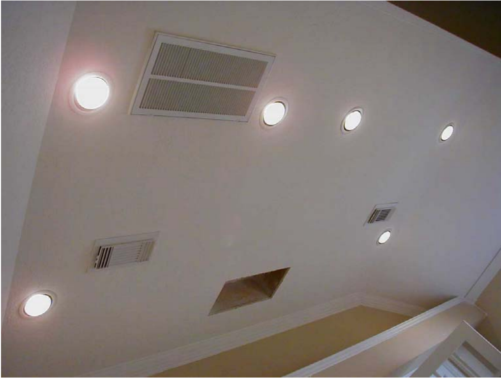
Photograph 3: Ceiling penetrations in a cathedral ceiling
