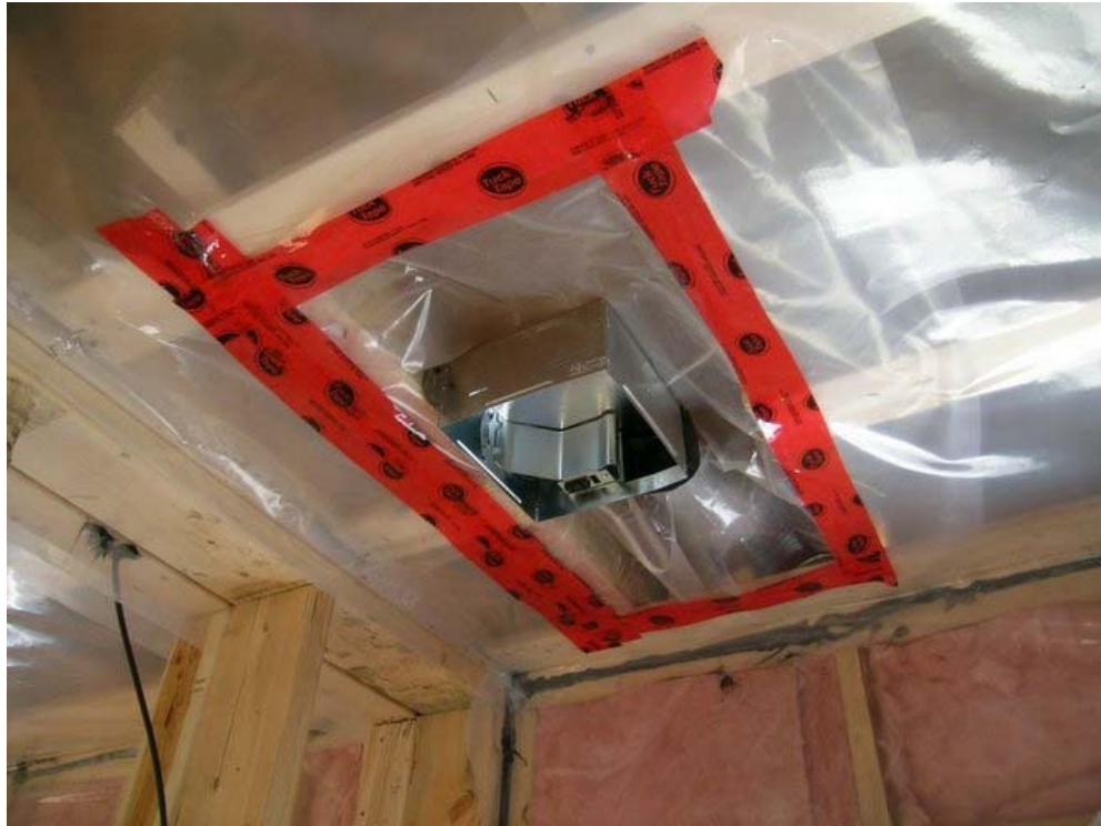
Photograph 4: Polyethylene sheet sealed as air barrier around bathroom fan housing
