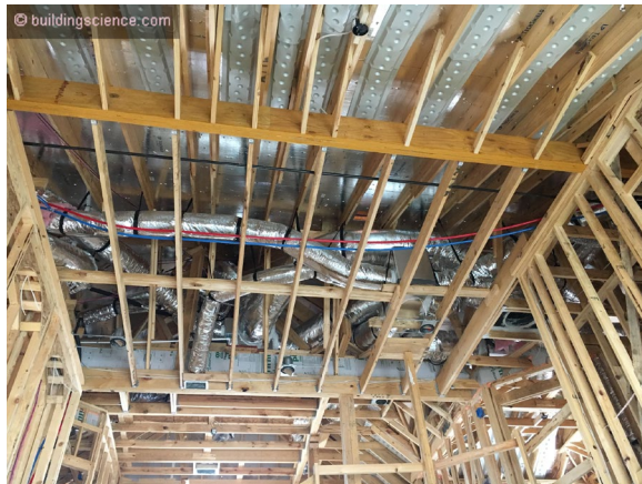
Photograph 5: Radiant Barrier in Attic - Once attic insulation goes above R-30 radiant barriers provide little or no benefit. Note that the current International Energy Conservation Code calls for minimum attic thermal resistance of between R-38 and R-60.
