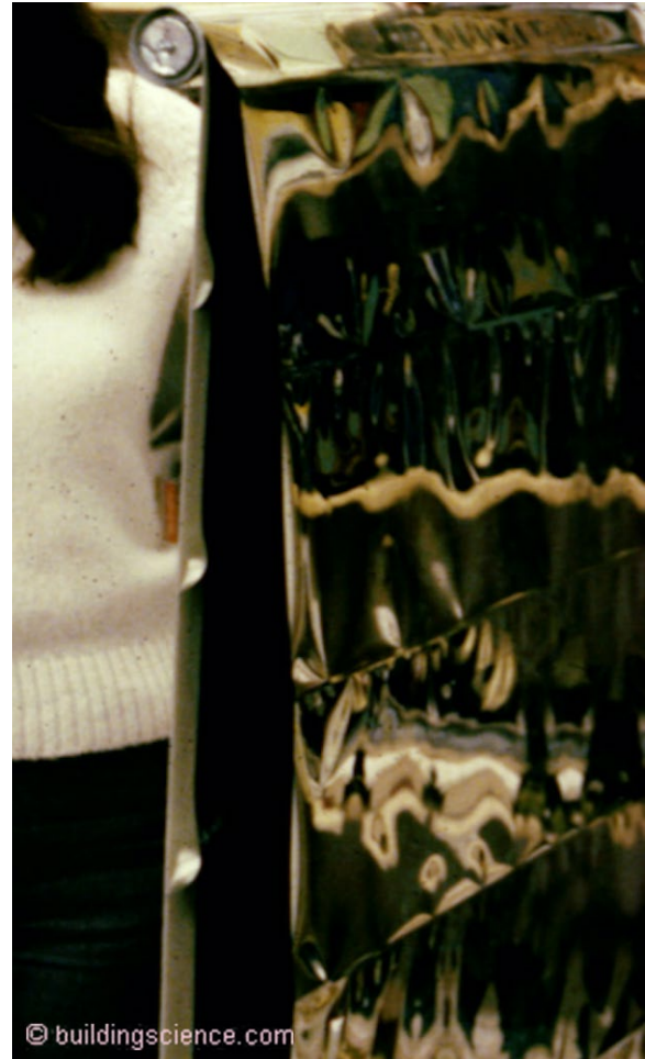
Photograph 3: Reflective Insulation Roll Blinds - The blinds 4 layers expanded as they were pulled down creating 4 airspaces each about 1 inch deep. Unfortunately there was no practical way of air sealing the airspaces. R-15 sounded great to me. I was young. Queen had a hit song “Another One Bites the Dust”. I didn’t realize it was about the thermal performance of the roll blinds.
