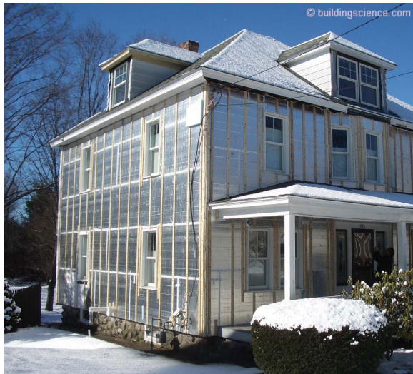
Photograph 6: Exterior Aluminum Foil - What I like about the aluminum foil on the exterior face of the exterior continuous rigid insulation is that it is a great water control layer, air control layer and vapor control layer. It also gives a big boost to the structural integrity of the rigid continuous insulation. So yeah to all that....but to say it gives a big boost to wall assembly R-value...slim to none....
