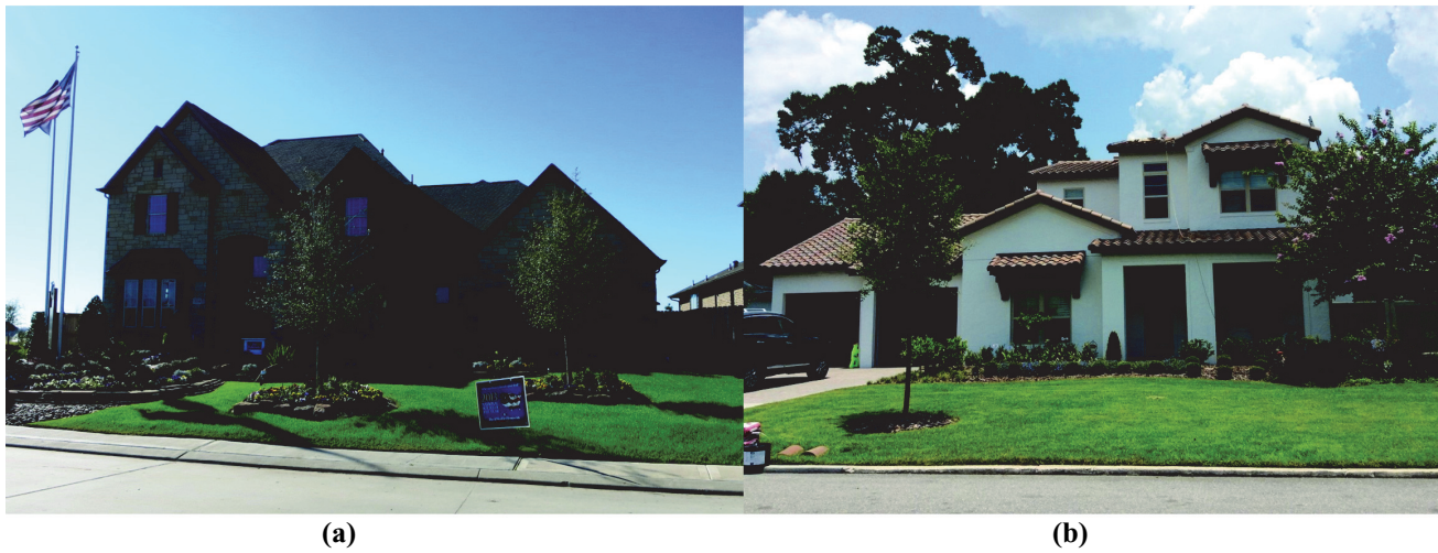
Figure 2 Front views of (a) Houston, north elevation, and (b) Orlando (west elevation) test roof houses.
