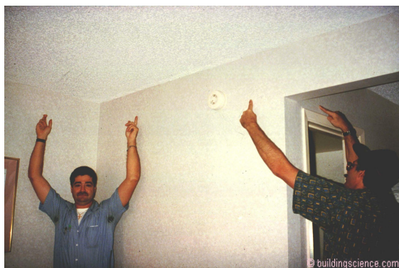
Photograph 8: Interstitial Negative Pressure Field - The negative pressure field of the bathroom dropped ceiling is coupled to the bathroom/hotel room wall...which is then subsequently connected to the hotel room demising wall which then extends outward to the exterior.
