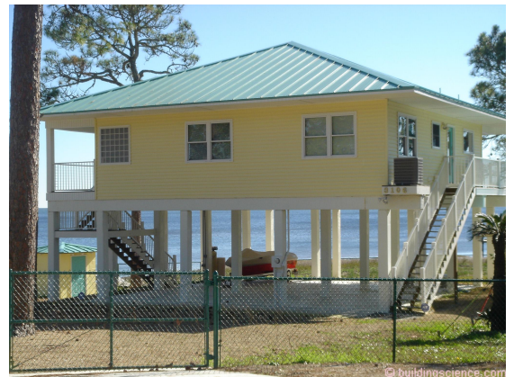
Photograph 3: Raise heating, ventilation and cooling (HVAC) equipment above the Base Flood Elevation (BFE) to prevent damage.
