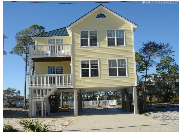
Photograph 2: In coastal areas the first level should be used for parking and storage.
