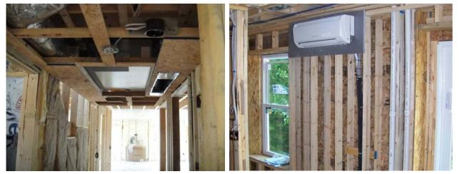
*Figure 2* Minimally-ducted mini split mounted in dropped ceiling space (left) and single-point wall-mounted ductless split indoor unit (right)
