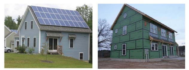
*Figure 1* Completed house example (left), and house under construction, showing exterior air barrier approach (adhesive tape sealed seams on exterior sheathing) (right)
