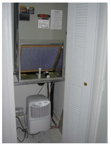
Photograph 6: Part Load Humidity Control: Individual dehumidifiers are provided in each unit – typically in the air handling closet – to handle part load humidity in hot humid climates.
