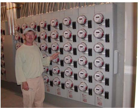
Photograph 4: Individual Metering of Services: Rational behavior is encouraged when all services are metered and billed separately.
