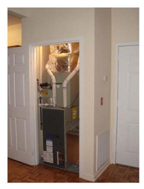
Photograph 1: Space Heating: Sealed combustion gas furnace provides space heating.
