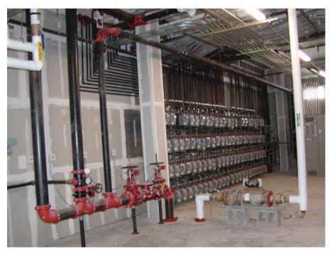
Photograph 5: Individual Gas Metering: Gas for space heating and domestic hot water is separately metered to each individual unit.
