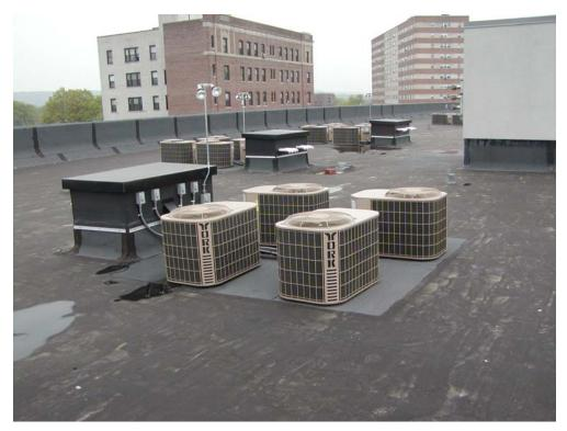
Photograph 3: Services Located on Roof: Rooftop penetrations are collected and located in "doghouses" – all cable, duct and pipes are run through walls of "doghouses".
