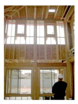
Additional savings could be realized by redesigning the wall with a single upper beam supporting the roof above the upper windows
