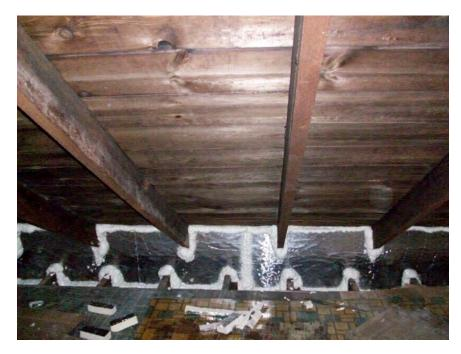
Figure 5. Foil-faced polyisocyanurate insulation board with seams and joints sealed to adjacent framing
