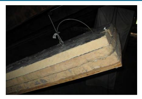
Figure 14. Hinged attic hatch with counterweight over attic access stairs. Gaskets and weather stripping are located on the stationary frame.
