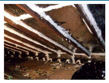
Figure 6. Foil-faced polyisocyanurate insulation board between roof rafters and transitioning to top of wall with seams and joints to adjacent framing sealed
