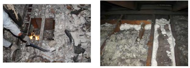
Figure 9. Left: Creating access to dropped soffit area and plumbing wall; Right: Attic floorboard repurposed in sealing plumbing chase (Photo credit: S. Marchese, printed with permission)
