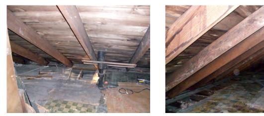
Figure 3. Left: Attic floorboards removed to investigate conditions at top of wall during assessment of prototype house; Right: Attic floorboards removed to allow access to top of wall
