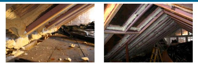
Figure 25. Left: Extruded polystyrene and wood furring strip used to extend rafter cavity; Right: Attic with rafter cavities extended in preparation for mineral fiber insulation (Photo credit: S. Marchese, printed with permission)
