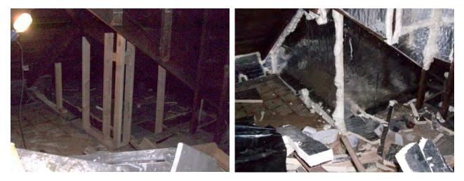
Figure 20. Left: Framing added above exterior wall at inset entry; Right: rigid board insulation installed to transition thermal control from exterior wall to roof assembly
