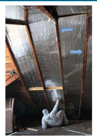
Figure 23. Foil-faced polyisocyanurate insulation fit into rafter framing cavities (Photo credit: S. Marchese, printed with permission)
