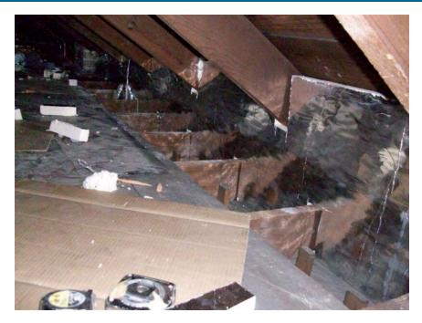
Figure 4. Foil-faced polyisocyanurate board insulation installed to transition thermal control from top of masonry wall to roof. The rigid insulation board rests on top of a wood plate at the top of the brick wall. Note that furring cavity gap (at junction of wall plaster and ceiling plaster) is to interior side of the rigid board insulation as indicated by wood furring extending above the top of the brick wall.
