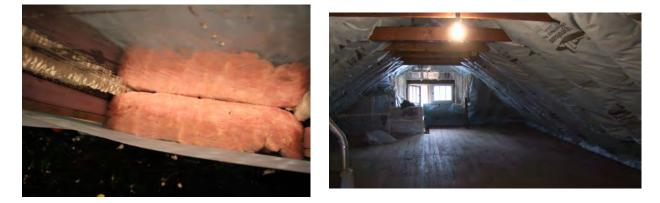
Figure 26. High density fiberglass batt in extended rafter cavity; Right: Completed roof rafter strategy (Photo credit: S. Marchese, printed with permission)
