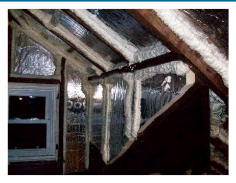
Figure 24. Foam sealant applied to seal foil-faced polyisocyanurate to surrounding framing. In this image the application of rigid insulation and foam sealant is not complete. (Photo credit: E. Haber, printed with permission)
