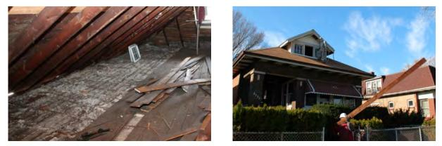
Figure 8. Left: Attic floorboards partially removed for attic deck air sealing and insulation; Right: Attic floorboards removed intact (Photo credit: S. Marchese, printed with permission)
