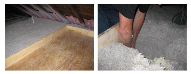
Figure 16. Left: Attic storage platform with insulation dams at the perimeter; Right: A CEDA Weatherization team member checks the depth of insulation beneath platform
