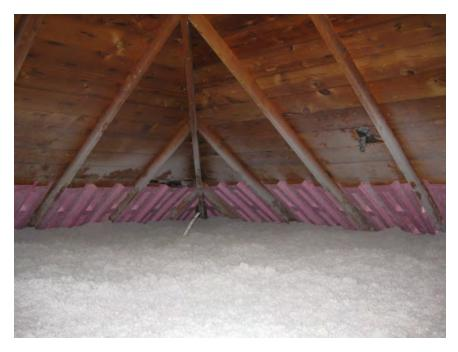
Figure 17. Vent chutes used to block cellulose from filling roof soffit
