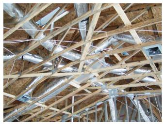
**Photograph 1: Ducts in Vented Attic** – At least they are shiny. What are the odds that they are tight? Good luck with that.
