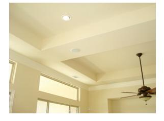
**Photograph 4 (at left): Soffit for Ductwork and Services** – Changes the appearance. Sometimes folks like it, sometimes not.
