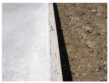
**Photograph 4: Thermal Break**—A thermal break worthy of great artisans. Install a strip of waterproofing set in mastic that spans the rigid edge insulation that acts as both a capillary break and an insect barrier.
