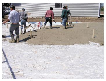
**Photograph 3: Concrete Placement**—Shows concrete being placed on the top of the sheet polyethylene and a layer of XPS insulation. Notice that there is no welded-wire mesh. Stones – gravel keep the plastic from blowing away.
