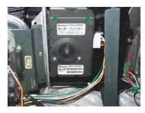
integrated supply ventilation system includes the installation of a Carrier cooling system with a 2-stage compressor, an ECM indoor fan motor, and a Thermidistat controller. The 2-stage compressor allows better matching of the load to the cooling system capacity to avoid poor humidity control inherent with short-cycling of over-sized systems. The electronically commutated motor (ECM) allows lowering the flow rate of air over the cooling coil for enhanced moisture
