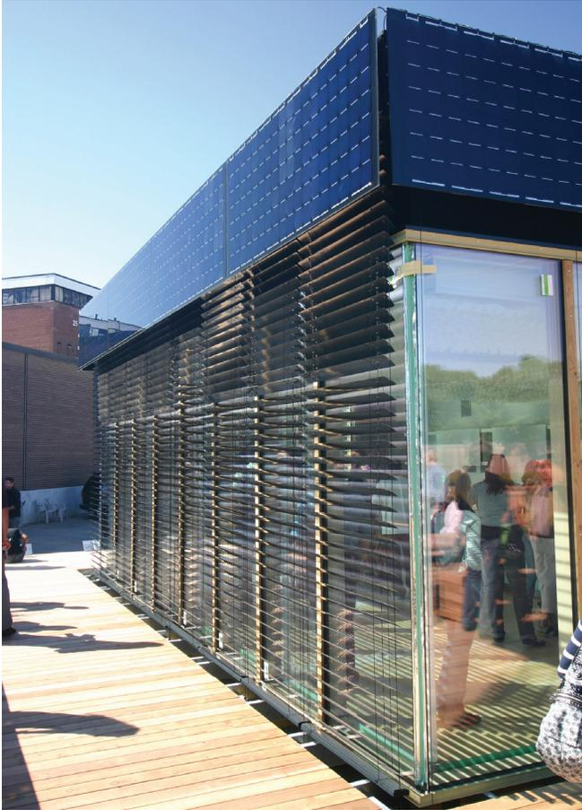
Figure 2. Quad-pane high r-value glazing and insulated wood frames, with operable exterior shades.
