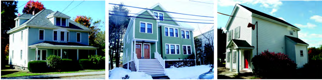
Figure 2 Front views of case study houses (left to right): Concord Four Square, Arlington Duplex, and Bedford Farmhouse.
