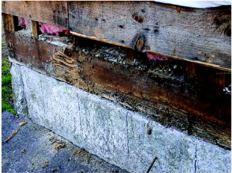
Figure 7 Sill detail, including air barrier transition wrapped to front of foam, and capillary break over foundation (left); existing sill beam, showing long-term moisture damage (right).
