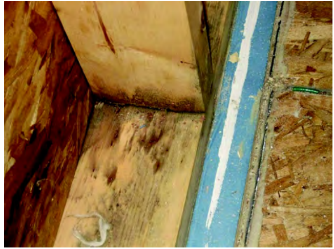
Figure 18 Moisture on bottom plate.
