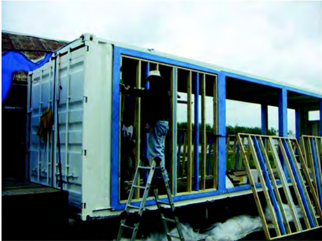
Figure 1 Installation of specimen wall framing in container.
