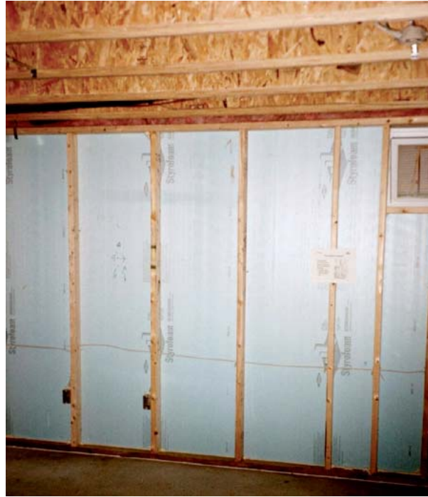
Figure 2 - Exterior Walls 2" x 6" Studs 24" Stud Spacing
