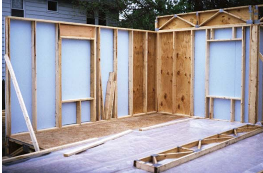
Figure 6 - Exterior Walls Non-Load Bearing Headers Removed
