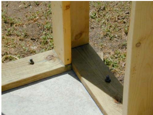
Figure 3 - Exterior Walls 2-Stud Corners
