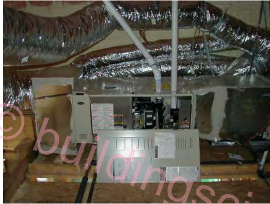
Figure A-6a. Photograph of air handler unit of two-stage compressor with ECM fan and Thermidistat system
