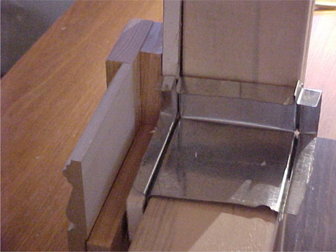
This picture clearly shows the air path behind the trim and the drywall detail. This system provides ~23 square inches of free air space.
