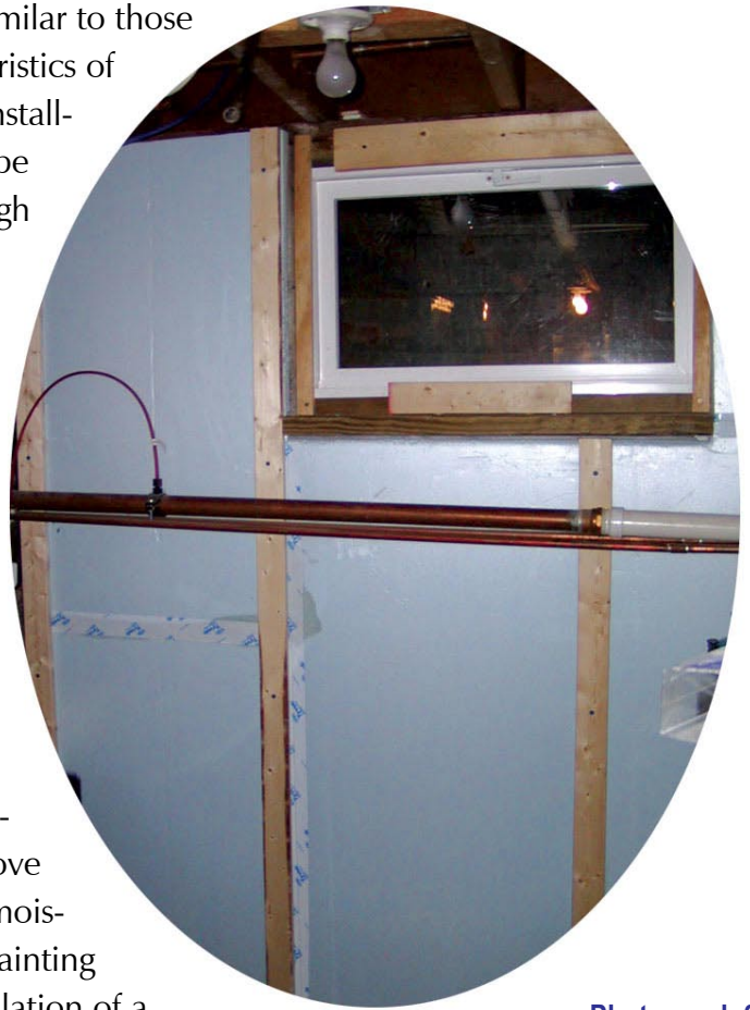
Photograph 2 XPS against basement wall with furring strips
