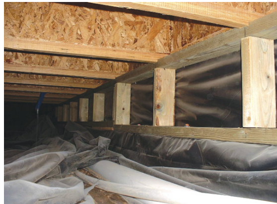
Figure SC-7: Conditioned crawlspace
