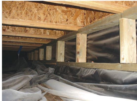
**Figure SC-7:** Conditioned crawlspace
