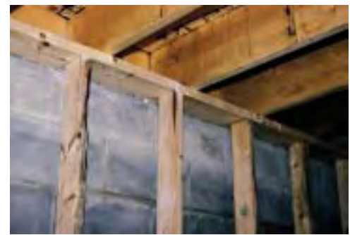
Photograph 1 Interior stud framing located at basement perimeter
