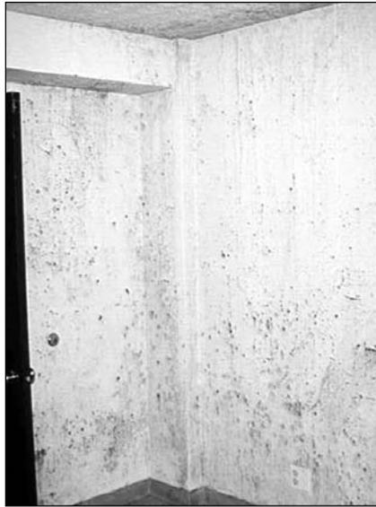
Mold growth on exterior walls was one of the most visible symptoms of moisture problems at this Cleveland Housing Authority apartment.
