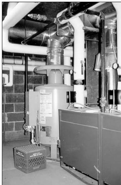
The new boiler and domestic water heater at West Broadway helped to improve apartment temperature control.
