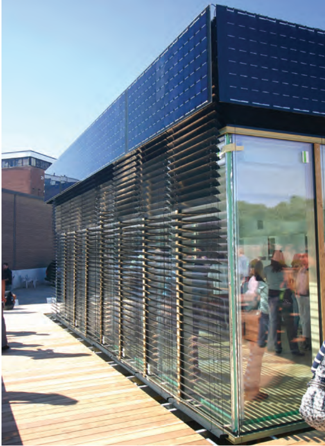
Figure 2. Quad-pane high r-value glazing and insulated wood frames, with operable exterior shades.
