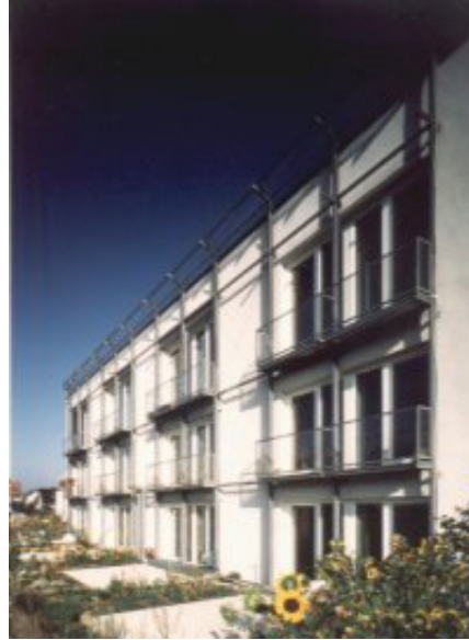
Passive House in Darmstadt, Kranichstein - South elevation (left) and interior (right) (From http://www.passiv.de/ )
