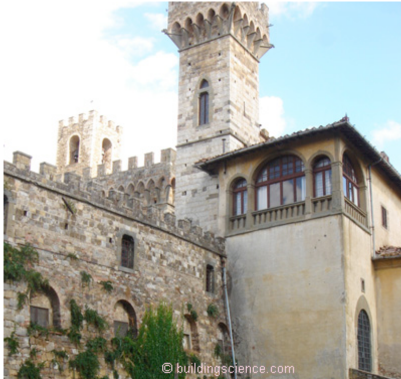
Photograph 1: French Chateau -A nice place to store wine is in its cellar.
