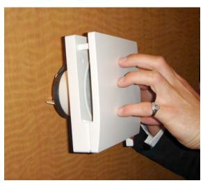
Photograph 4 (above left): Weather-Stripped Door—A beautiful thing if you are worried about fires – an ugly thing if you need make-up air. Photograph 5 (above right): High Tech Big Hole—Good for about 25 cfm, so you need three or four per apartment. They diffuse the incoming air to avoid cold spots and drafts.
