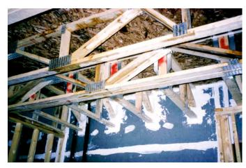
Photograph 1: Compartmentalization Air Sealing—Gypsum board is run up to the underside of the floor sheathing above and sealed with joint compound.
