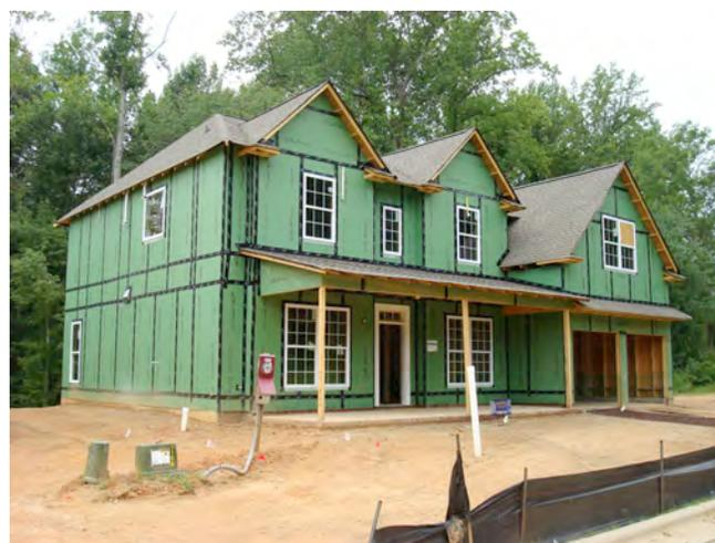
**Photograph 1: OSB Water Control Layer** – OSB where the water control layer is integral with the OSB sheathing where taping the joints provides water control layer continuity.
