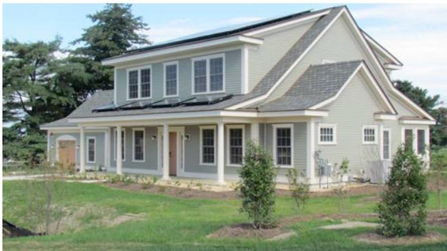
**Photograph 3: Completed Ultra Tight House** – Looks like any other house, just tight and ventilated right. Balanced fully ducted heat recovery ventilator with sealed combustion appliances and powered make-up air when air consuming appliances are used. OK, it doesn't quite look like any other house because of the PV array and solar thermal stuff. This is the NIST Zero Energy Demonstration House in Gaithersburg, MD.
