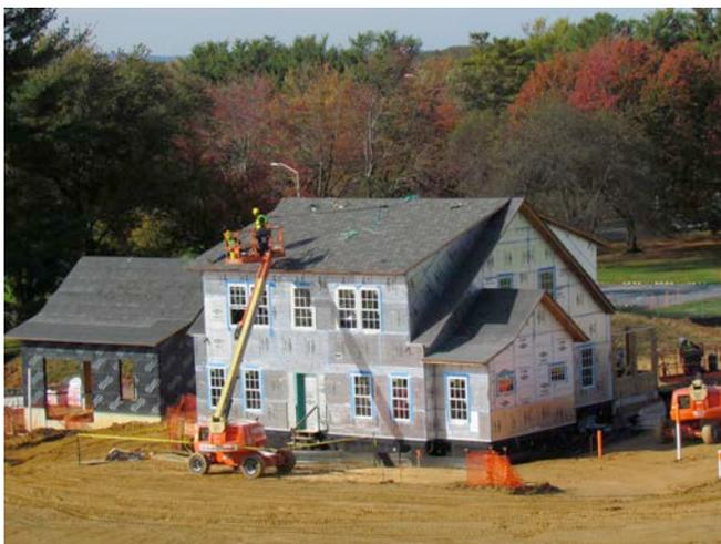
**Photograph 2: More Ultra Tight House** – Continuous exterior insulation installed over fully adhered exterior air control layer to control condensation at the exterior air control layer – structural sheathing interface. Note that the garage is not attached to the house. Good idea, but typically not possible.
