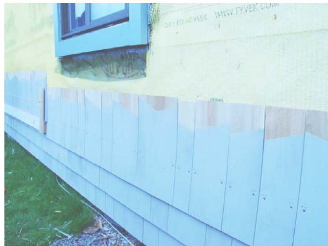
Photograph 2: Gap Behind Siding and Trim (left) —With wood and fiber cement siding and trim you need to install the siding and trim over a small gap to control hydrostatic pressure. This gap can be as small as a 1/4-inch and the spacer can be a strip of thin foam.
