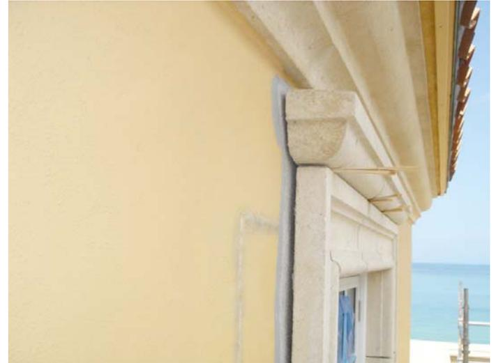
**Photograph 4: Precast Trim (above)**—It is absolutely critical to drain the back surfaces of these trim elements to prevent perched water and resulting hydrostatic pressure. There are countless sad stories of trim catching water at window to wall interfaces leading to wind driven rain driving forces in the absence of wind.
