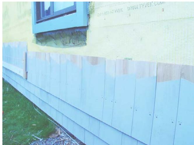
**Photograph 3: Drainage Mat (right)**—With cedar shingles you can use a drainage mat. You can also use a drainage mat with stucco – except you need to install building paper over the drainage mat so that it does not fill with the mortar from the stucco scratch coat.
