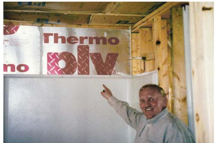
**Photograph 7: Tub on Exterior Wall After Tub Installation**—Notice the rigid material on the exterior wall behind where the one-piece shower/tub thingy is. Notice the even bigger smile on that VP of construction.
