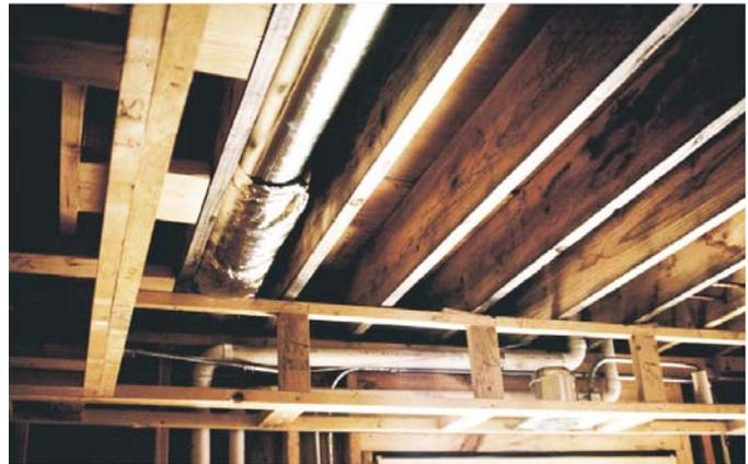
**Photograph 4: Soffit on Exterior Wall**—Wow, this allows for connecting your entire floor cavity to the outside.
