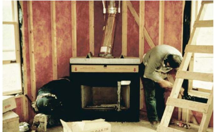
**Photograph 3: Fireplace on Exterior Wall**—OK, an even bigger hole than the bathtub hole. Kind of makes it funny to think about sealing an electrical wire going through a top plate when you have something this big.
