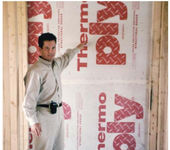
**Photograph 6: Tub on Exterior Wall Before Tub Installation**—Notice the rigid material on the exterior wall where the one-piece shower/tub thingy is going to be.
