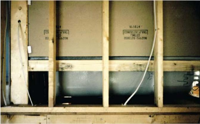
**Photograph 2: Bathtub on Exterior Wall**—The classic “Joe Hole”—a hole so big even I can crawl through it. It needs to be draftstopped with something rigid and airtight. Note to folks out there in the real world: fluffy insulation is not rigid and airtight. But a sheet of OSB or gypsum board over fluffy insulation makes the fluffy insulation happy and Joe happy.
