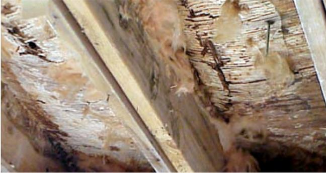
**Photograph 10: Condensation and Decay are Bad**—Air permeable insulation under deck can lead to condensation and decay. You would never construct an unvented roof this way. So why would you ever construct a deck this way?
