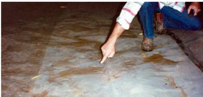
**Photograph 6: More Crawlspace Condensation**—How did the water get on the top of the plastic ground cover? It condensed out of the ventilation air.
