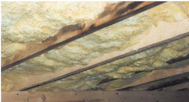
**Photograph 5: Crawlspace Condensation**—Water droplet forest on underside of crawlspace subfloor cavity insulation.
