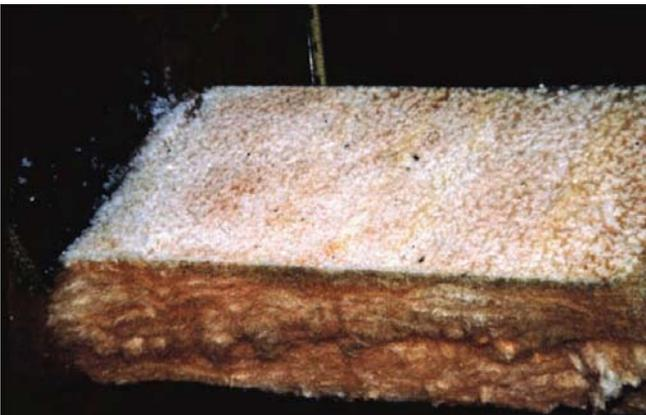
**Photograph 7: Radiation Coupling in Attic**—Frost on the top surface of attic ceiling insulation.
