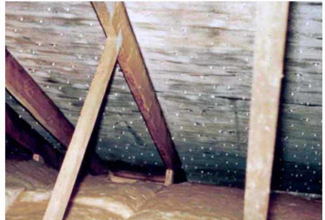
**Photograph 3: Roof Sheathing**—Nails frost up first, then the underside of the roof sheathing.
